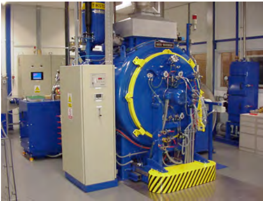
Figure 6. Seco/Warwick Vacuum Furnace
